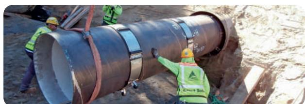
Steel line pipes are used in transmission pipelines in the oil and gas, and water and sewage sectors. The line pipes are also used as piles at ports and jetties
